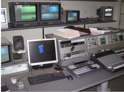
Broadband intake (first floor)
